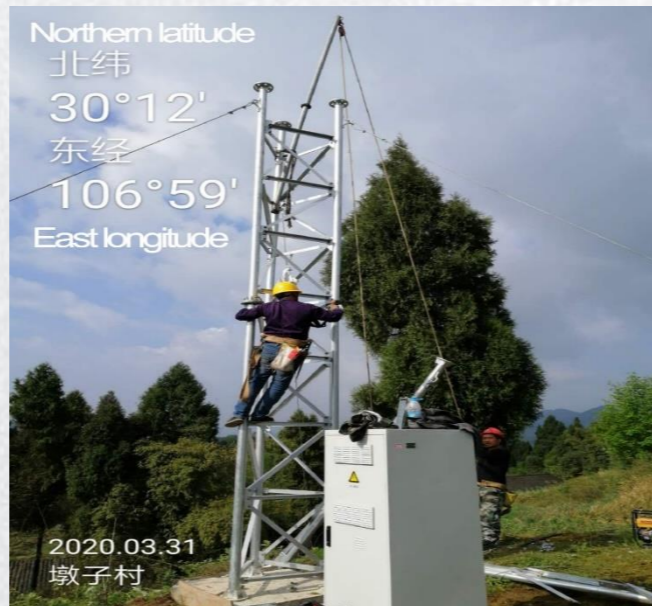
Lattice guy tower
