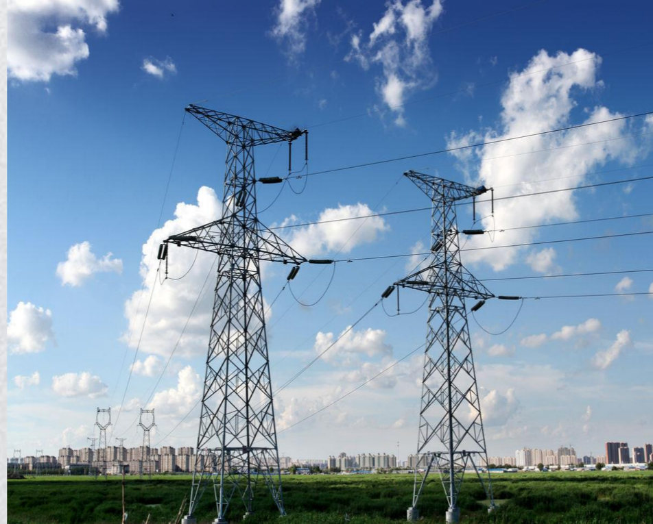
330Kv strain tower
