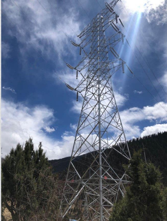
132Kv transmission tower
