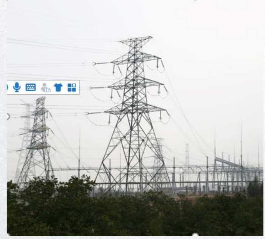
500Kv double-circuit tower
